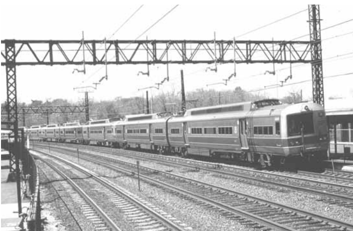
The catenary replacement project on the New Haven was complete when this photo at Rye, NY was taken in 2003.
