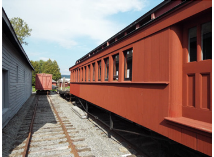
The Schoharie Valley Railroad Museum includes several buildings and rolling stock. Photo by Dave Hamilton.
