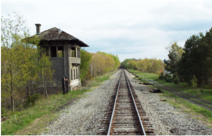
The 2018 KL&L Convention trip will include a visit to one of the former DL&W concrete interlocking towers.
