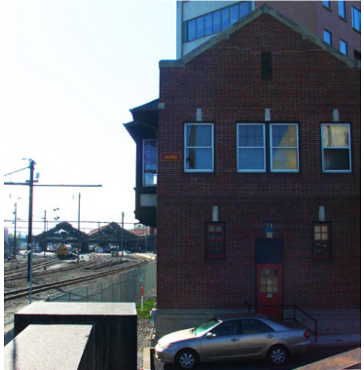
The restored Harris Tower offers a great vantage point to view action on the Amtrak and Norfolk Southern lines in downtown Harrisburg, PA. Photo by Dave Hamilton.
